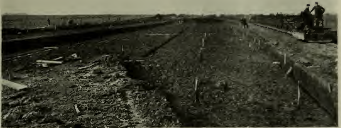
SHOWING THE PEAT ON WHICH PART OF THE REINFORCED CONCRETE ROADS AT MANCHESTER ARE BUILT.
